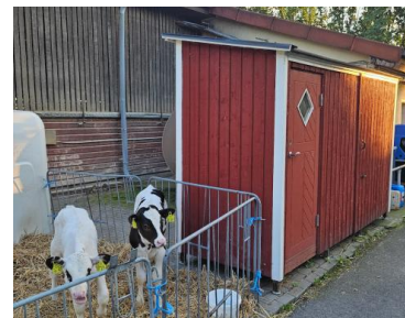
Figure 1: Solar house with solar pumping station, 1500L heat storage tank, and electrical
