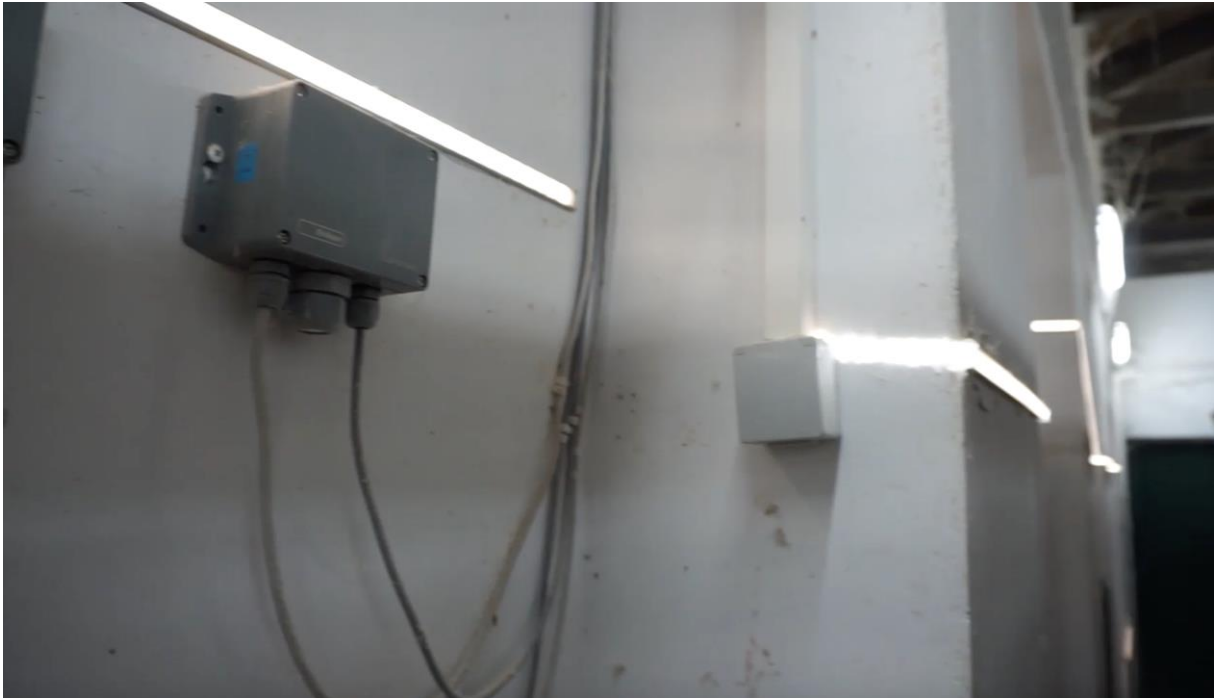
Figure 5. Figure 4. Snapshot from the RES4LIVE final video showing the LED lighting installation and smart controllers at AUA poultry farm, Greece.
