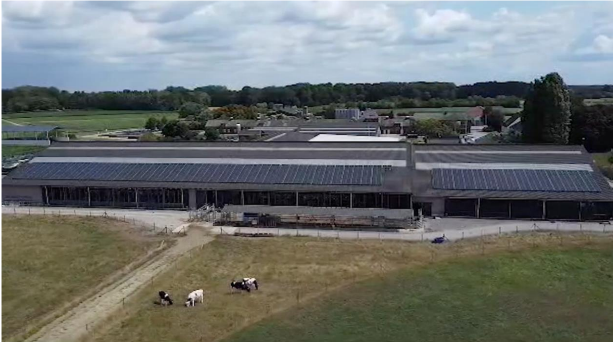
Figure 2. Snapshot from the RES4LIVE final video showing the PVT installation at ILVO swine farm, Belgium.
