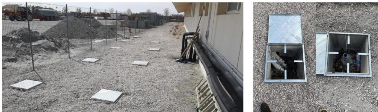
Figure 13. Restoration of the geothermal area and details of the pits: geothermal probe (left) and piezometer (right).
