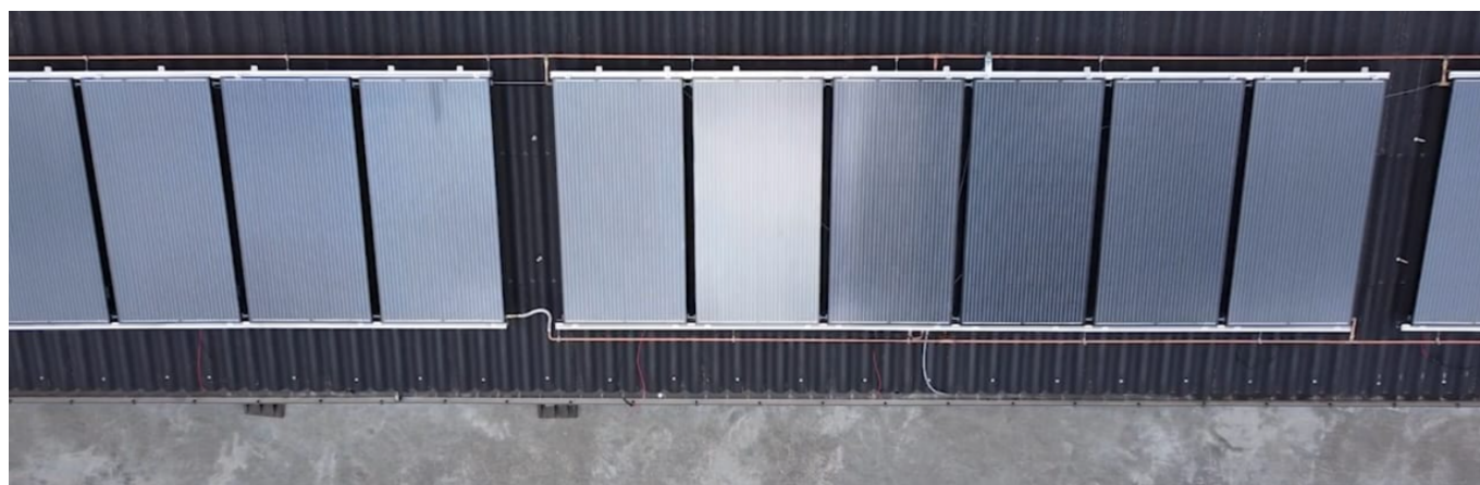
Figure 1: PVT collectors at ILVO swine farm in Belgium, before insulation of pipes
