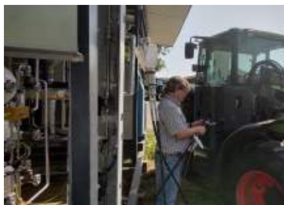
BioCNG upgrade plant and fillig station (left), filling up a CNG tractor (right)
